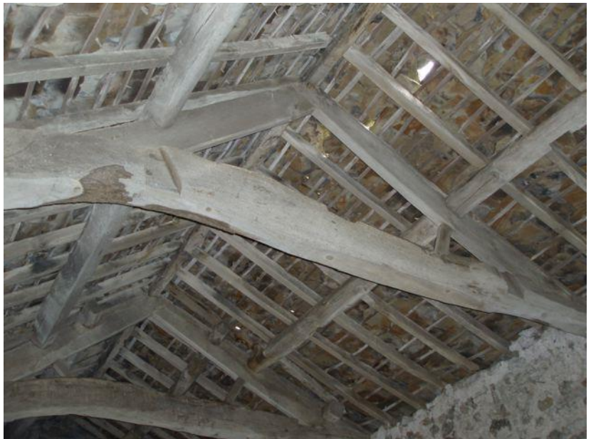
Figure 4 Renard Close Laithe: former cruck blades re-used in new roof trusses of 1667.
