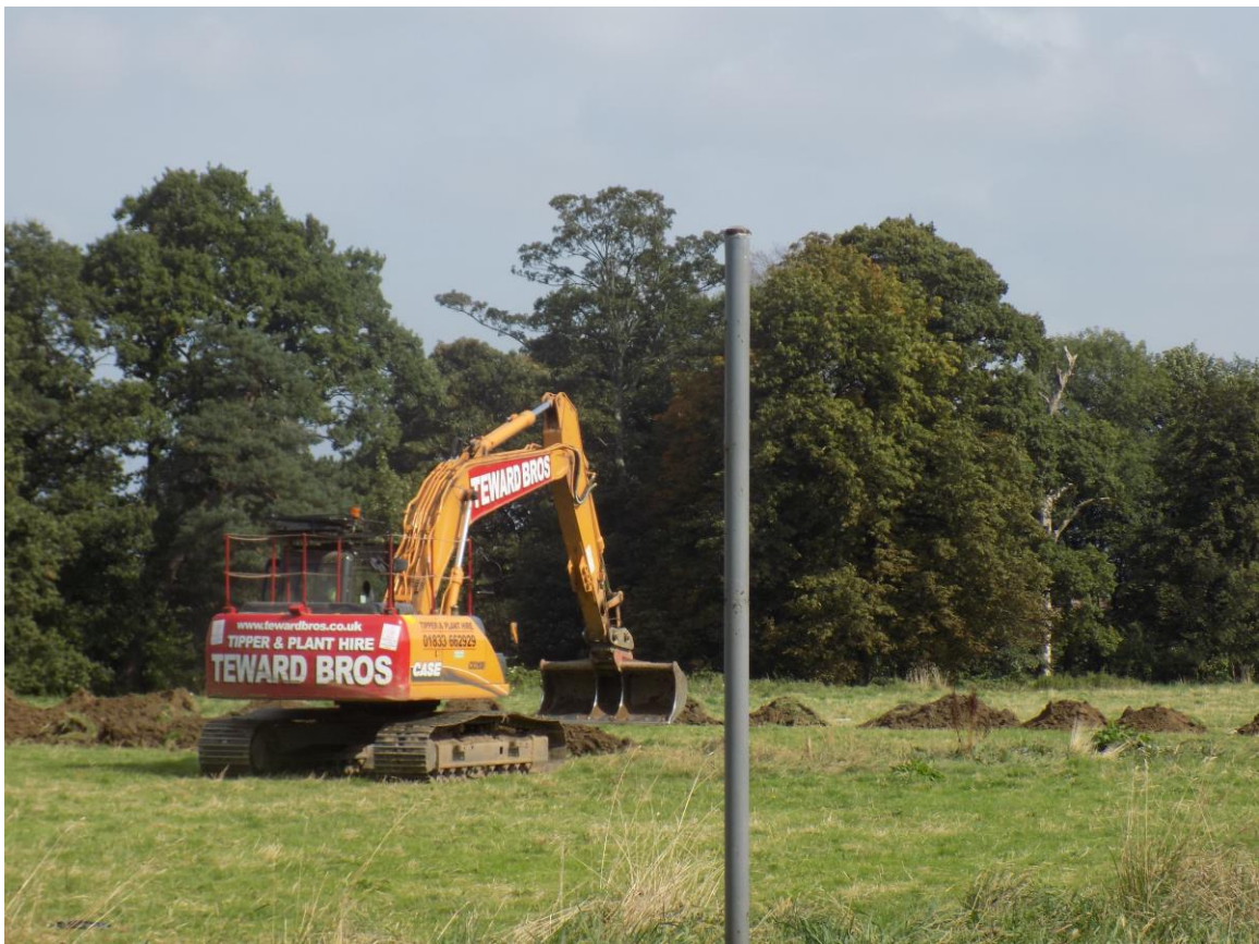
Hands On Middlesbrough's work brought increased scrutiny to bear on the Council's Acklam Hall site, where invasive ground works in sensitive areas commenced without suitable archaeological oversight. © Scarlet Pink.
