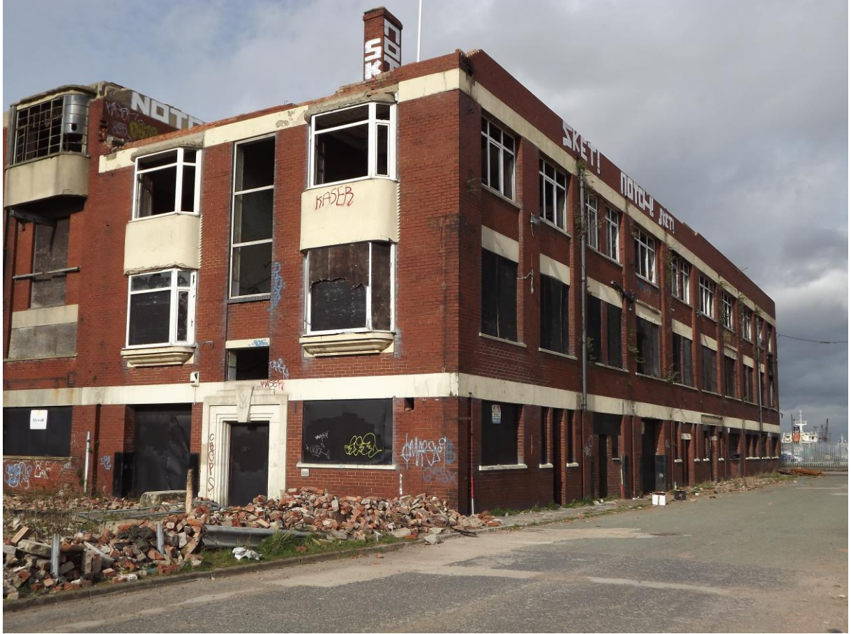
Figure 4 J Marr building, Kingston upon Hull.
