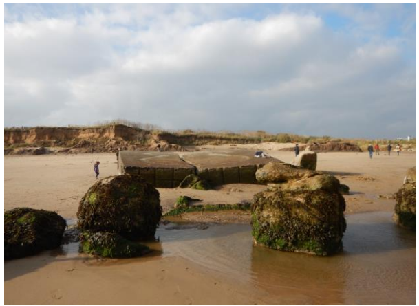
Figure 5 An eared pillbox destroyed by coastal erosion, the outline of its walls can be seen in the top of the foundation.
