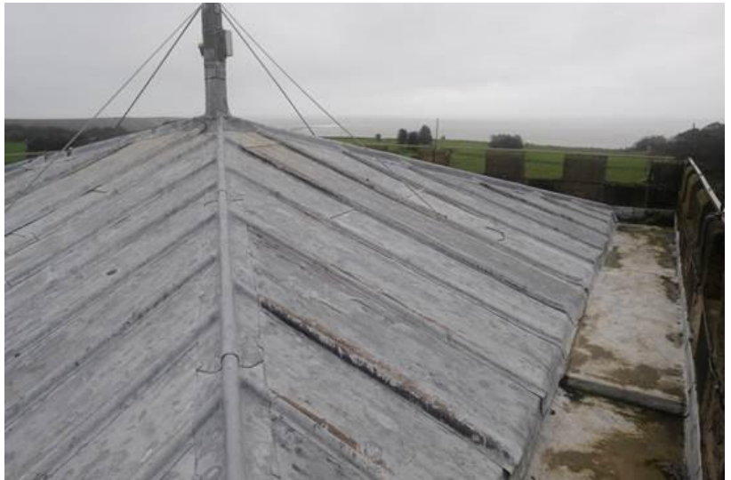
Figure 2 General view of the tower roof, looking east.
