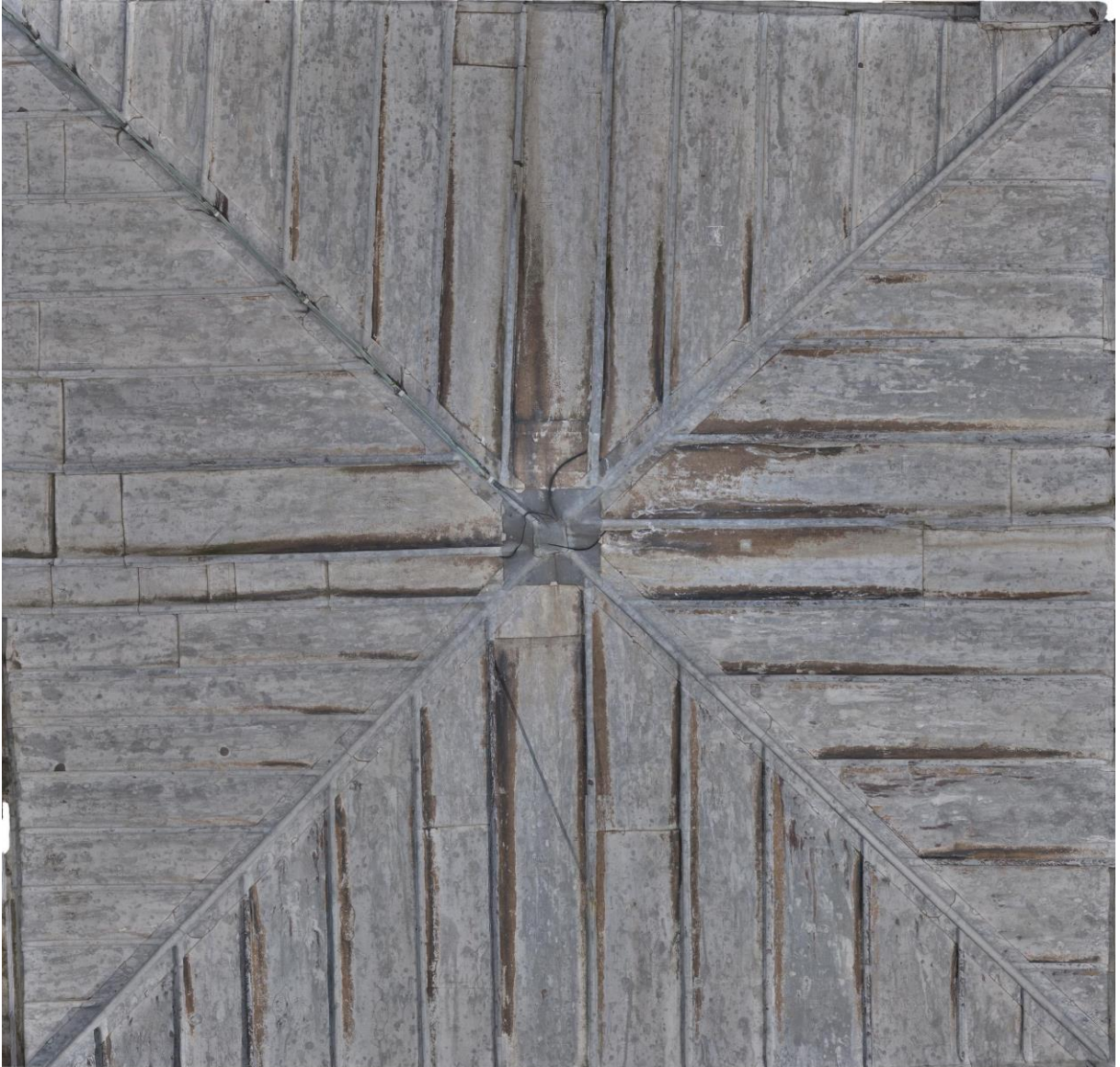
Figure 14 Ortho-rectified montage of St Oswald's Church roof generated from 1737 overlapping digital images. Image created by Nick Hannon © Historic England.
